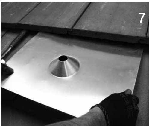
7 Cut a hole in the tile removed, with room to get the post through. Replace tile in position. Insert post and tighten into place. Install the 18" x 18" flashing, and apply sealant around the opening.
